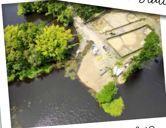
Desilting of Hillsborough Dam
