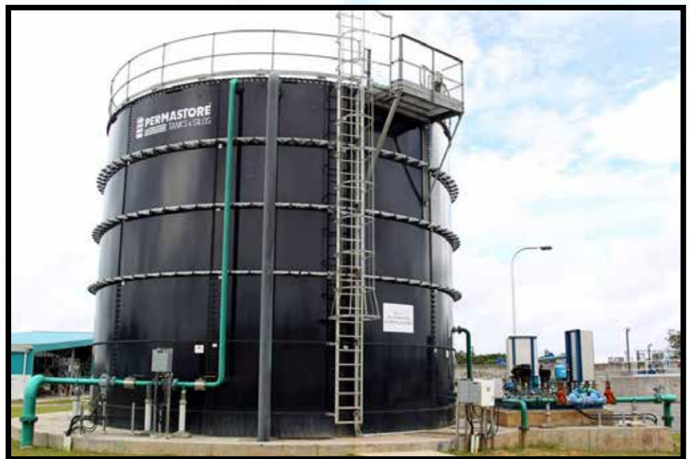
Tank at Malabar Wastewater Treatment Plant, Trinidad
